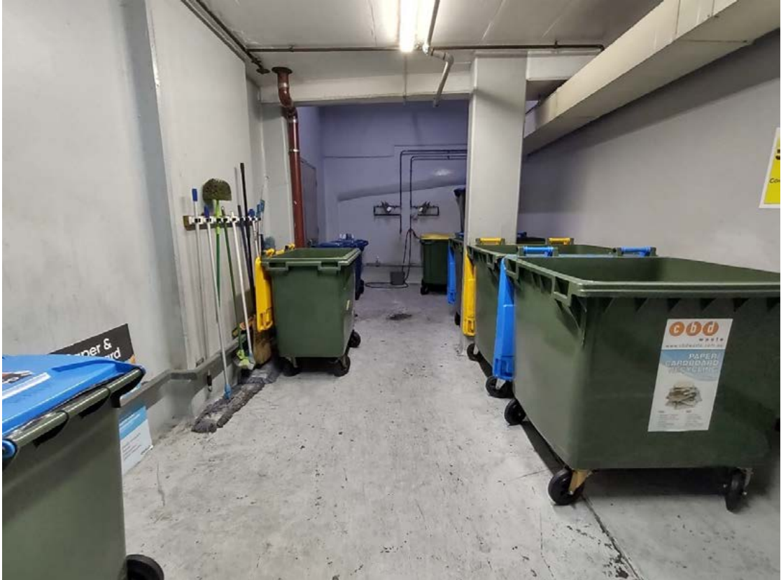
Photo 18: Recycled waste store room in basement 2
